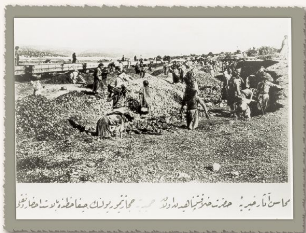
Construction Works of the Hedjaz Railways. Rail laying by local workers. Yıldız Saray Collection.
